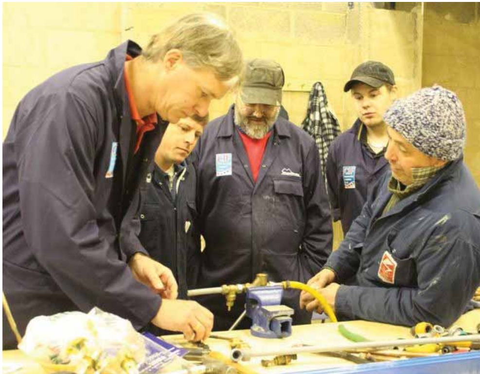
Simon Larkin (left) re-seating a tap under instruction from trainer, Jim Shearman (right)
